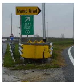
Figure 6 - An unmarked crash cushion in Republic of Croatia
