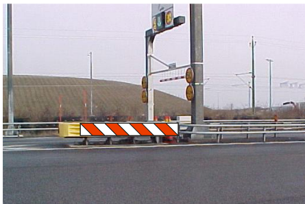
Figure 7 - Additional traffic marking of the crash cushions by signs K10 and K11
