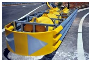
Figure 5 - Traffic marking of crash cushion in Republic of Croatia
