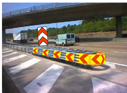
Figure 8 - The additional traffic labeling protective with cushions K8 and K14
