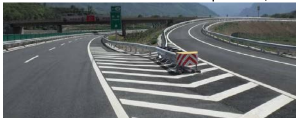
Figure 4 - Horizontal road marking in a place where crash cushion is installed
